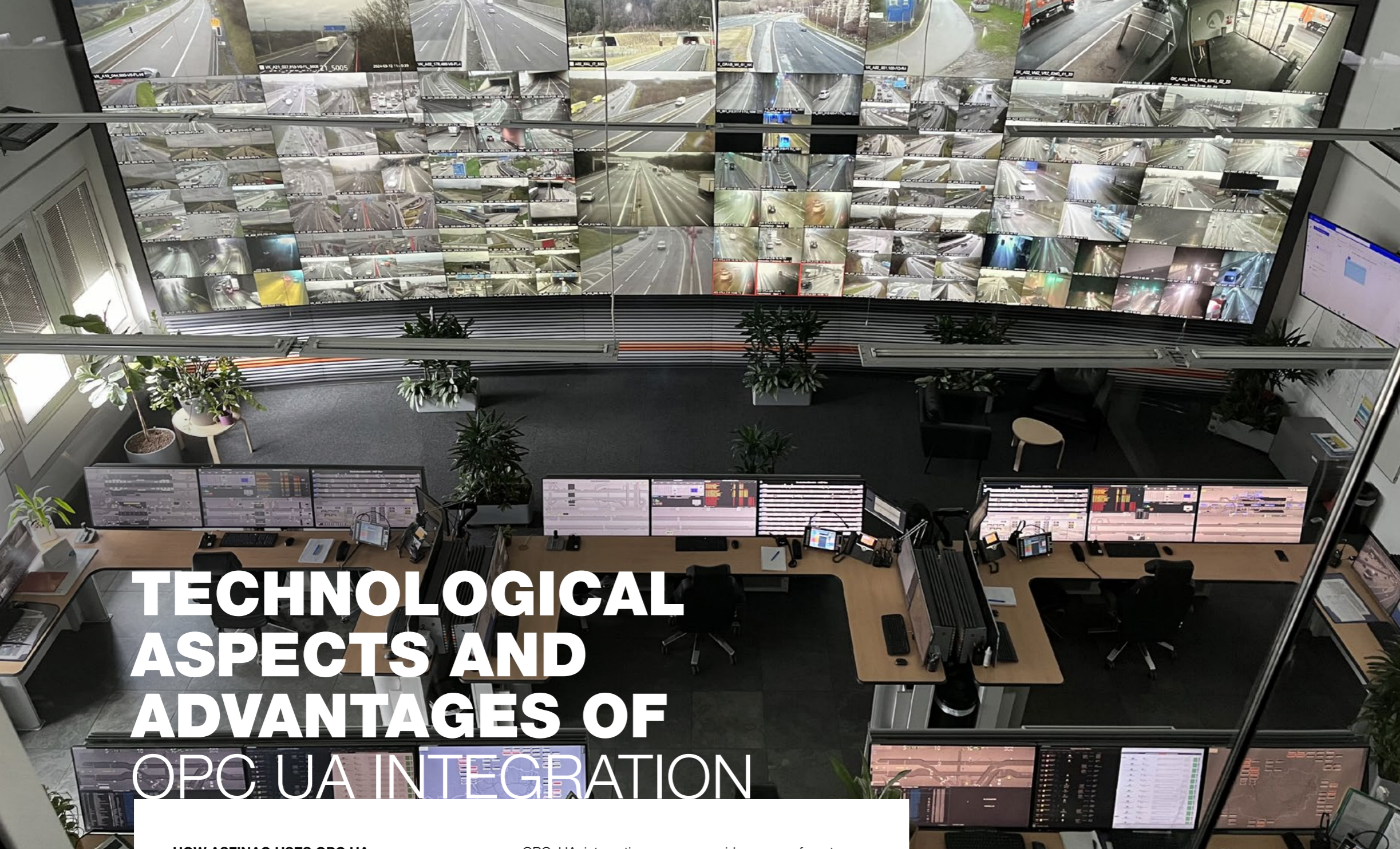
ASFINAG Traffic Management Center Vienna. © ASFINAG
